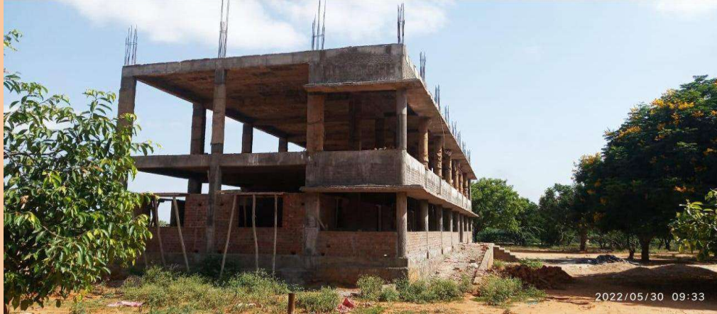
Construction of New Classrooms Block
